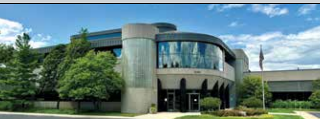
Our Global Headquarters in Waukegan, Illinois, U.S.A.
